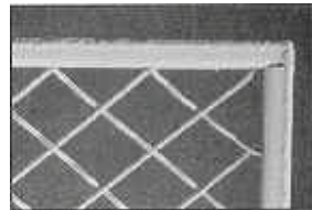
Figure 14: Welds may be undercut and may have pin holes
